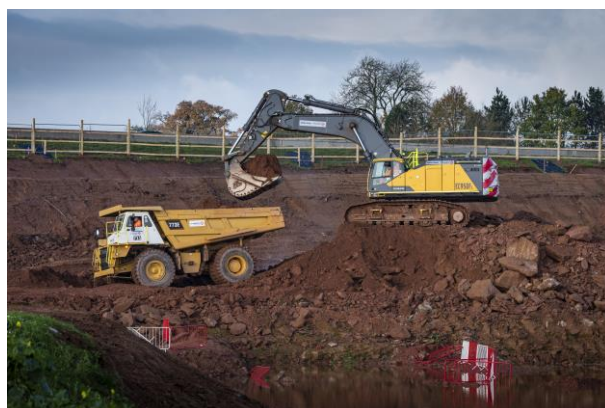
Progressing earthworks to build the box jack structure under the A46 by 2024
