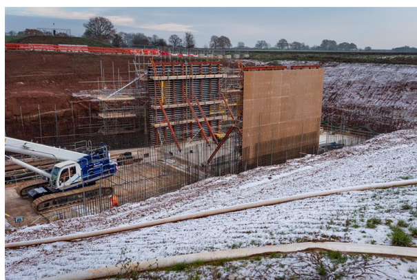
Constructing the box bridge for the Coventry to Leamington Spa rail Overbridge
